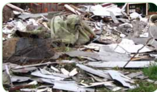
Broken asbestos cement materials from a demolition
