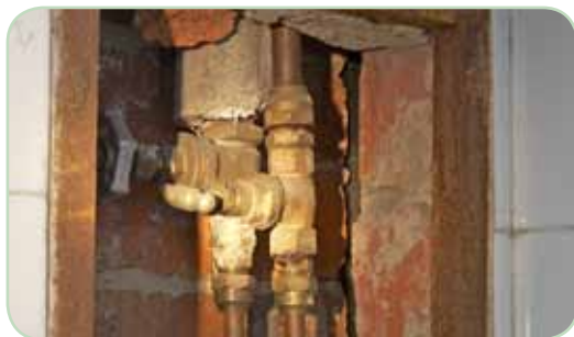
Friable asbestos lagging on pipes
