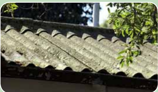
Asbestos cement corrugated roofing
