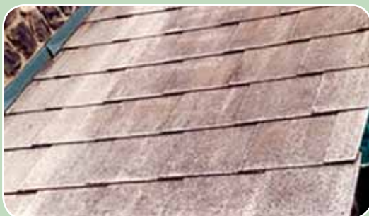
Asbestos cement shingles
